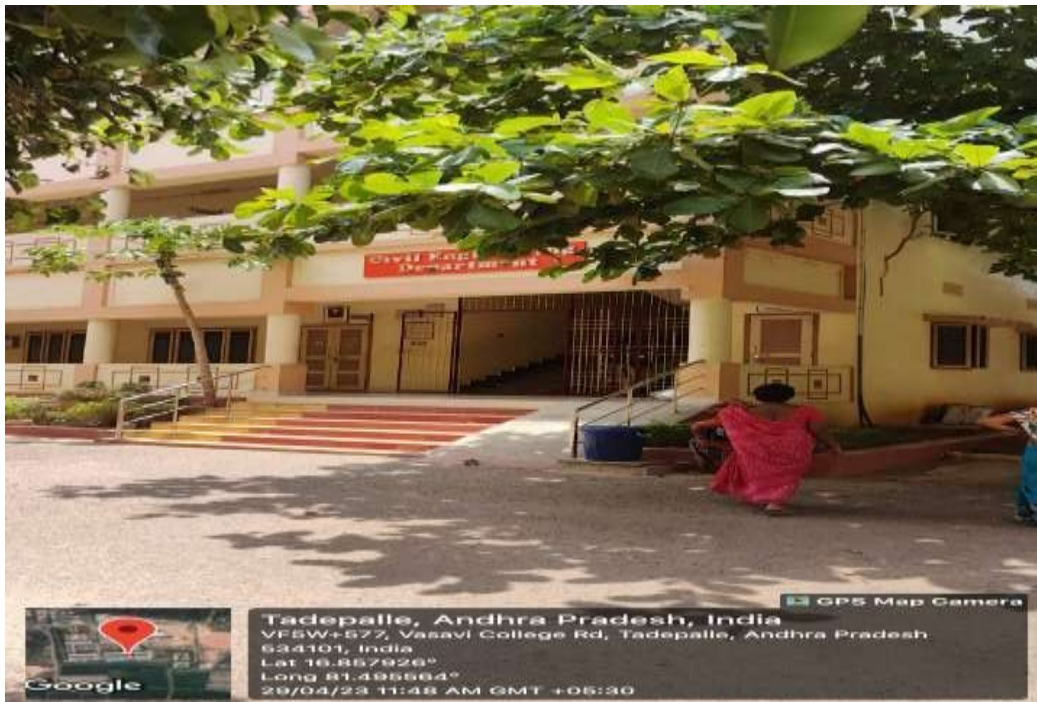
Civil Department ramp
