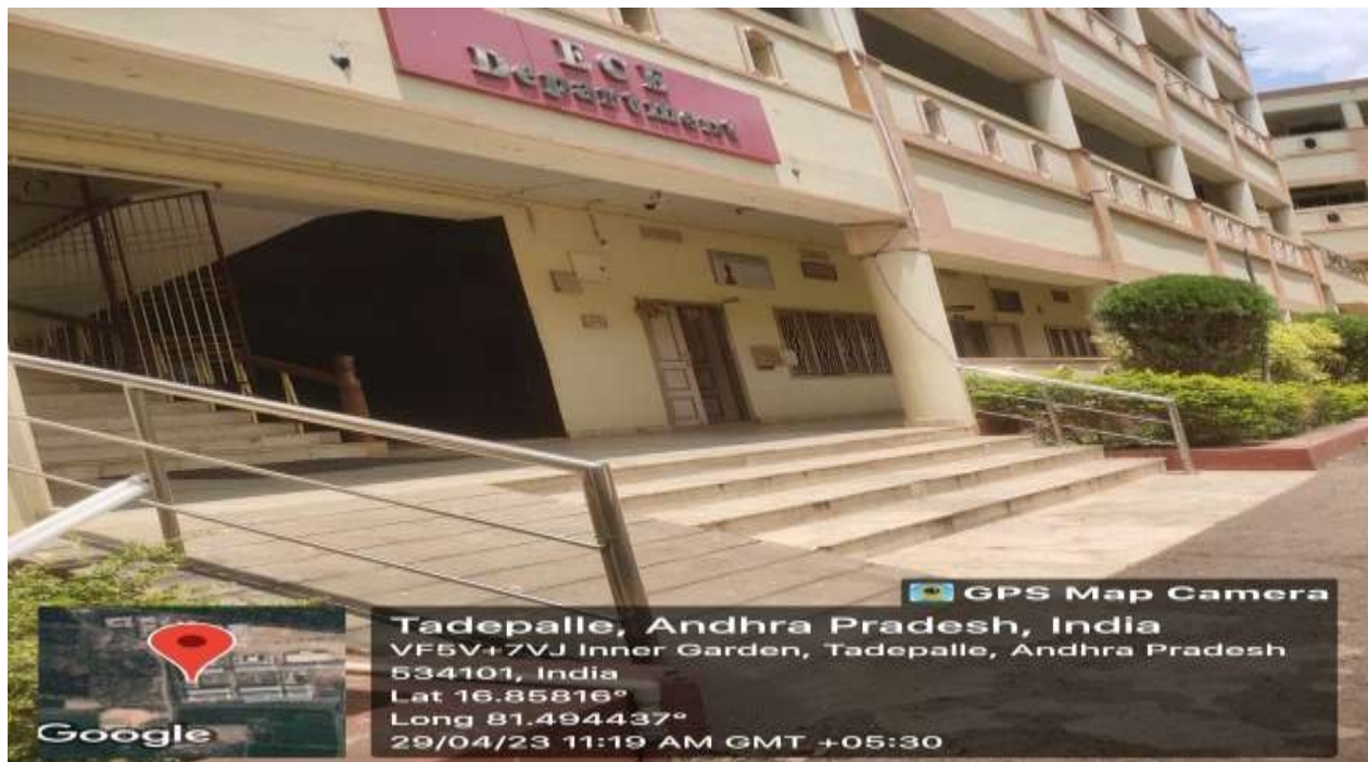
ECE Department ramp
