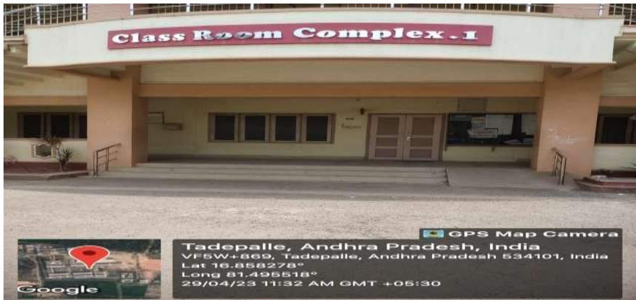
Class Room Complex with ramp
